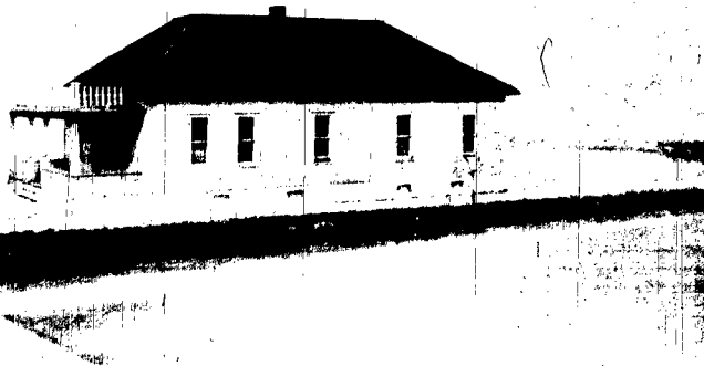
THIS IS THE WAYNE HOSPITAL that Dr. S. A. Lutgen started in Wayne years ago. It is no longer standing. At one time the hospital stood where Dahl's Retirement Center is now. This
